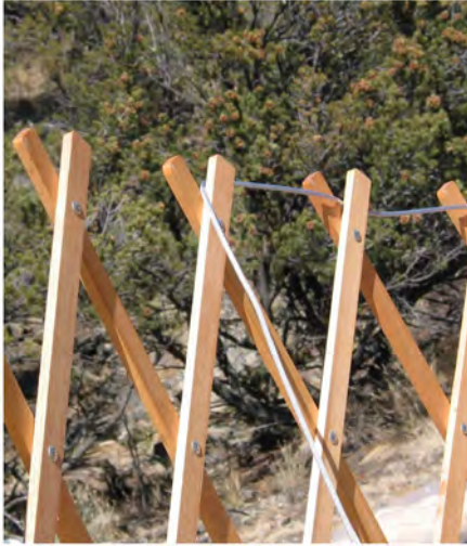
Cable rests on the top of the lattice wall.
