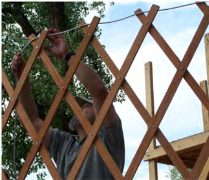
Cable rests on the top of the lattice wall.
