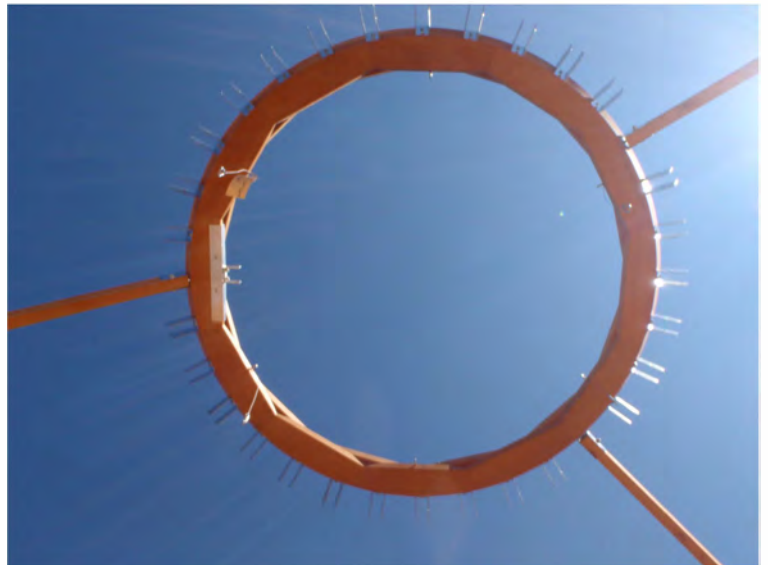
Compression ring is raised with 3 rafters. "Tripod method"
