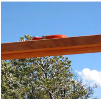
Cable hook on top of door frame.
