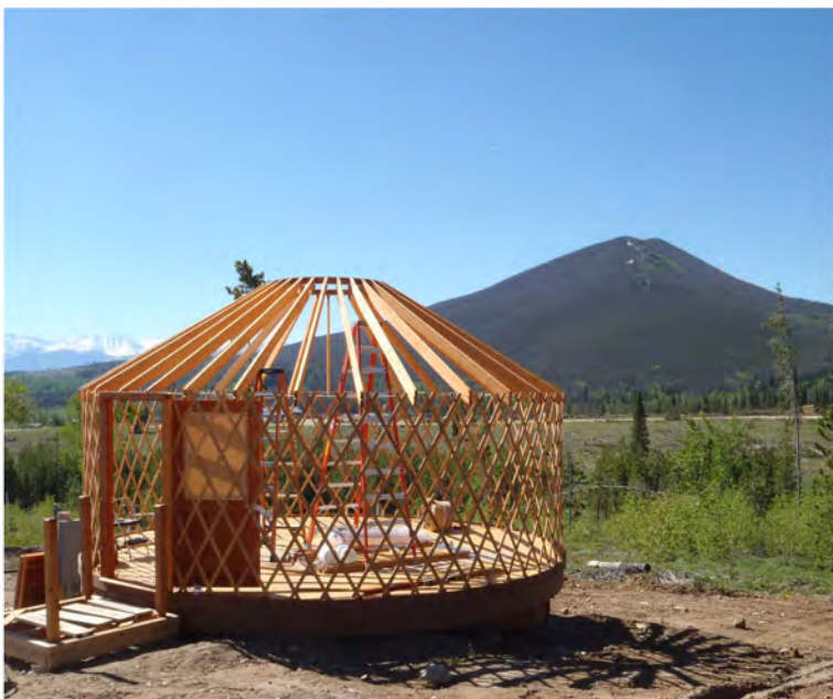
Entire yurt frame in place.
