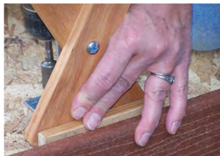
Steel brackets anchor lattice wall to deck.
