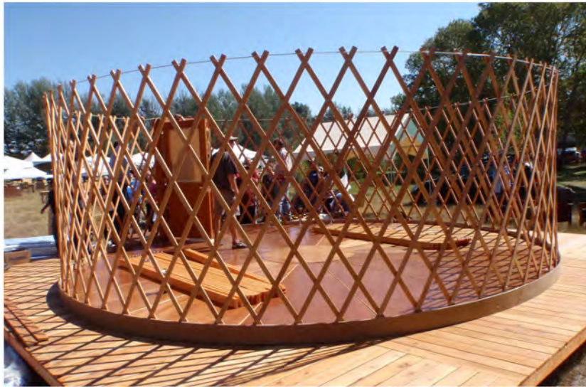
Lattice wall and door in place. Cable rests on top of lattice
