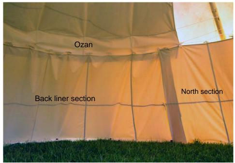
North section of liner overlapping the Back section, with ozan above
