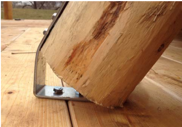
Steel bracket holds pole in place on deck (see price list for deck pitching kits)
